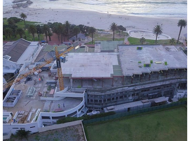
THE MARLY, CAMPS BAY · DURING CONSTRUCTION
