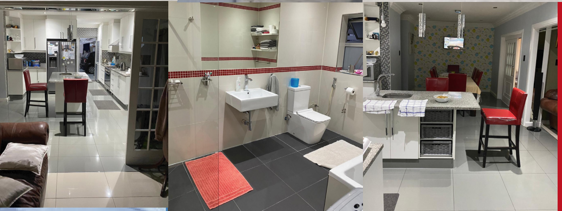
Complete renovation to Villa Alexander Location: Newfields
