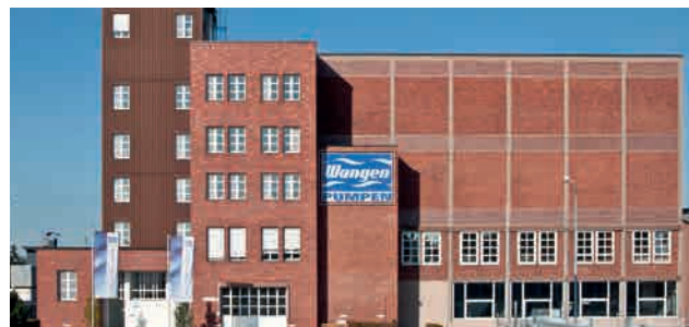
Headquarter building in Wangen
