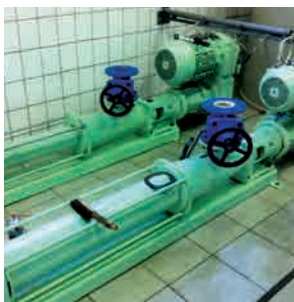
Conveyance of thin slurry: KL50S progressing cavity pump
