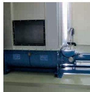
Conveyance of dewatered sewage sludge from decanter for drying: KL65R80.2 Triplex progressing cavity pump
