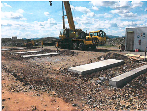
Concrete blocks 0,7m X 4,0m
