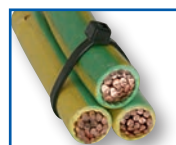
Nylon Cable Tie Tensioned/Cut/No sharp edges
