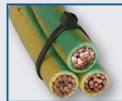
Nylon Cable Tie Tensioned/Cut/No sharp edges
