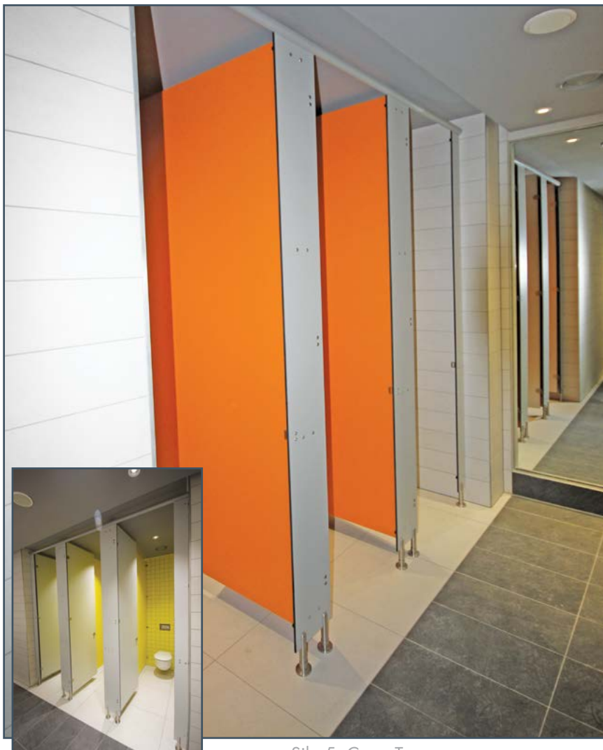
Silo 5, Cape Town
