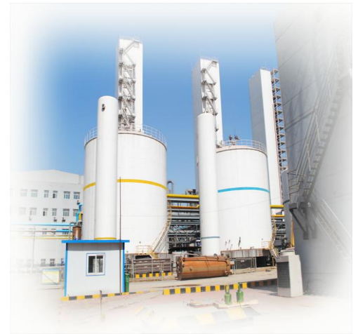
C. Liquid Nitrogen, Oxygen, & Argon Plant by Cryogenic Technology
