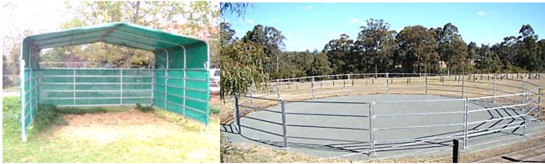
Shelter & Fence utilizing Economy Range Panels
