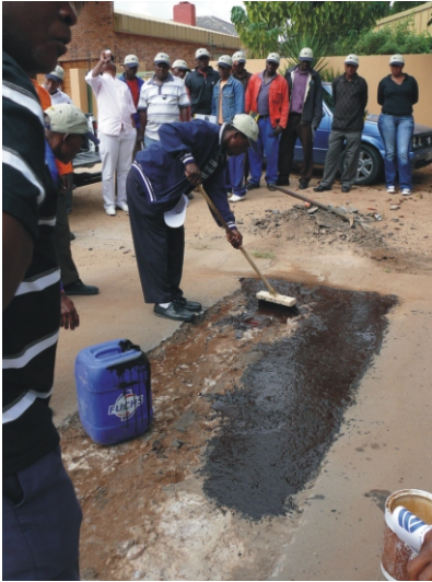
Applying primer on base using a stiff broom a
