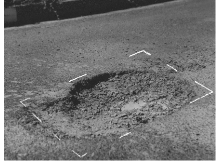
A typical pothole ready to be excavated along marked chalk line
