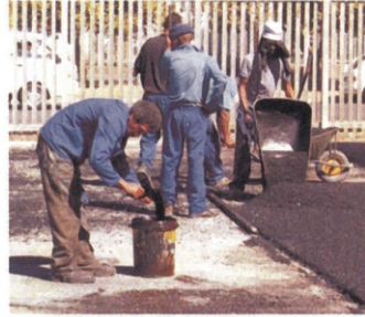
Applying tack by hand with a brush (turning area of a carpark)
