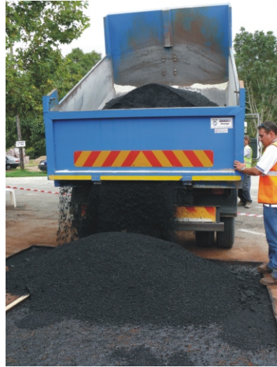
Tipping hot mix asphalt, ready for spreading
