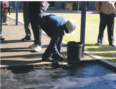
Applying primer to a joint before laying hot mix
