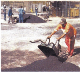
Barrowmen tip premix ahead of rakemen. Note close proximity of stockpile
