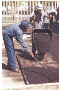
Rakeman spreads premix. Note the wooden gauge to achieve correct levels
