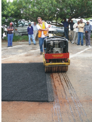
Compaction with a pedestrian roller.
