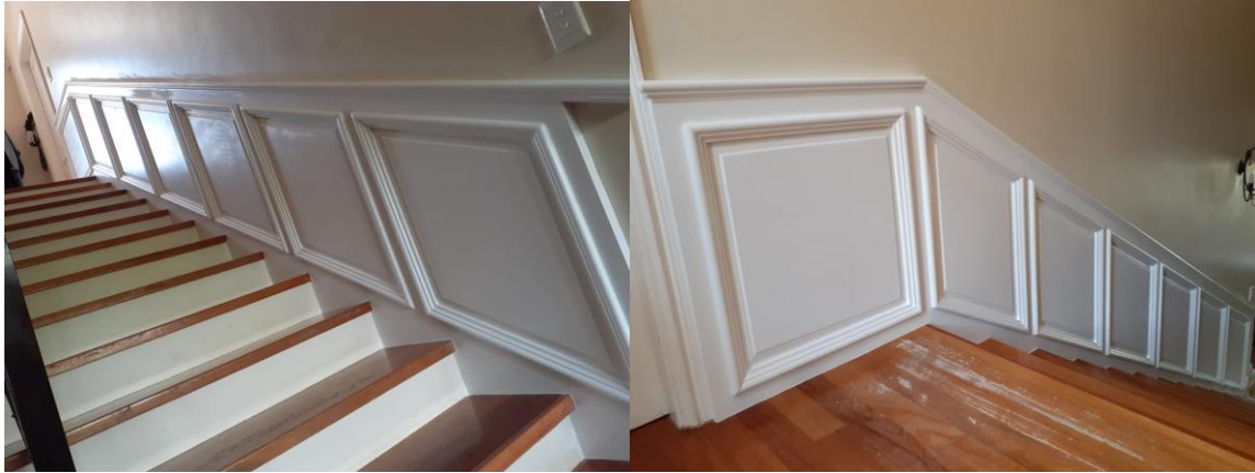
Supply of staircase cladding
